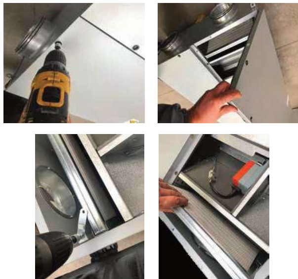
Filter replacement in the FLAT350 i FLAT550 model
